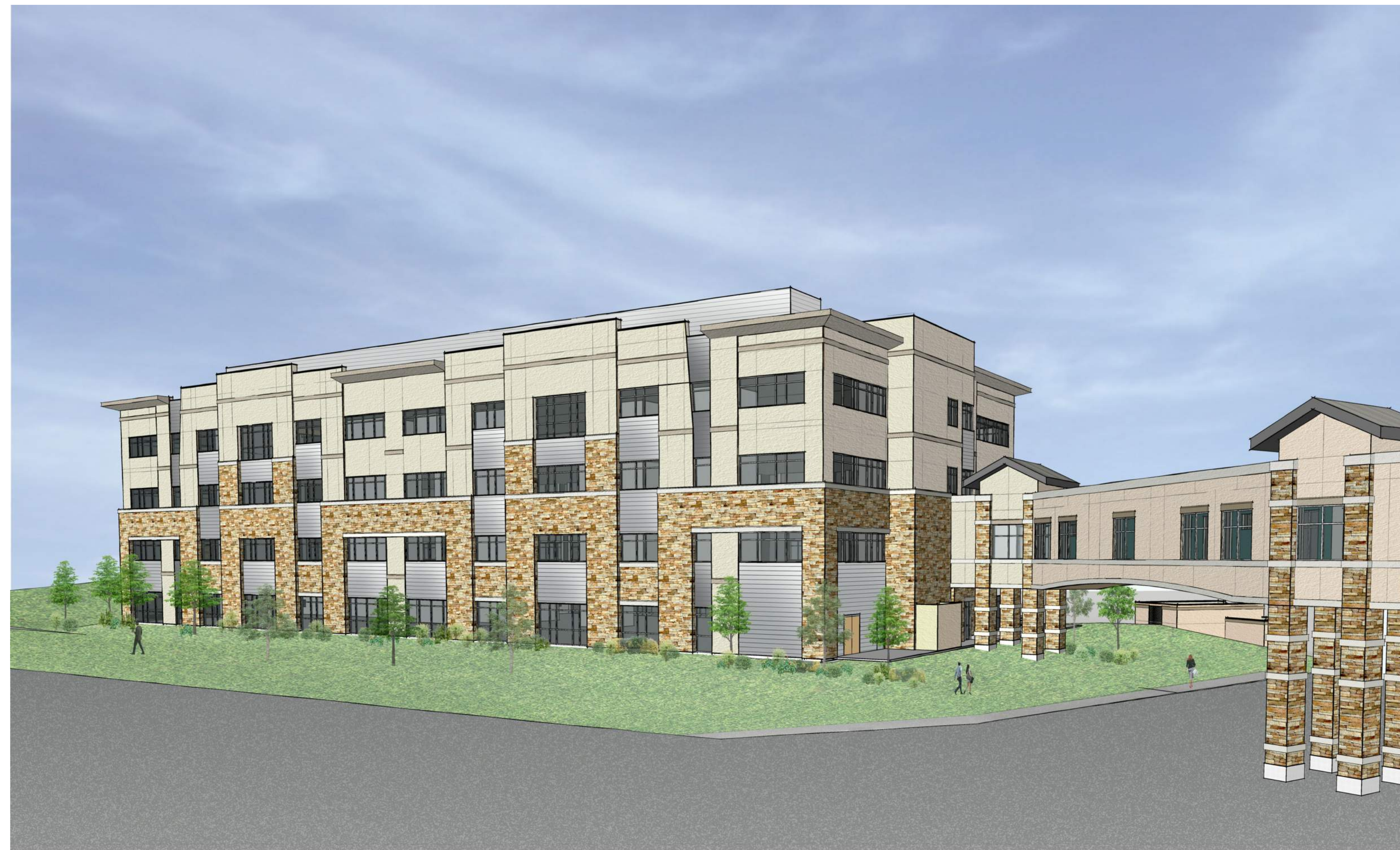
2 SP6 VIEW FROM NORTHWEST
