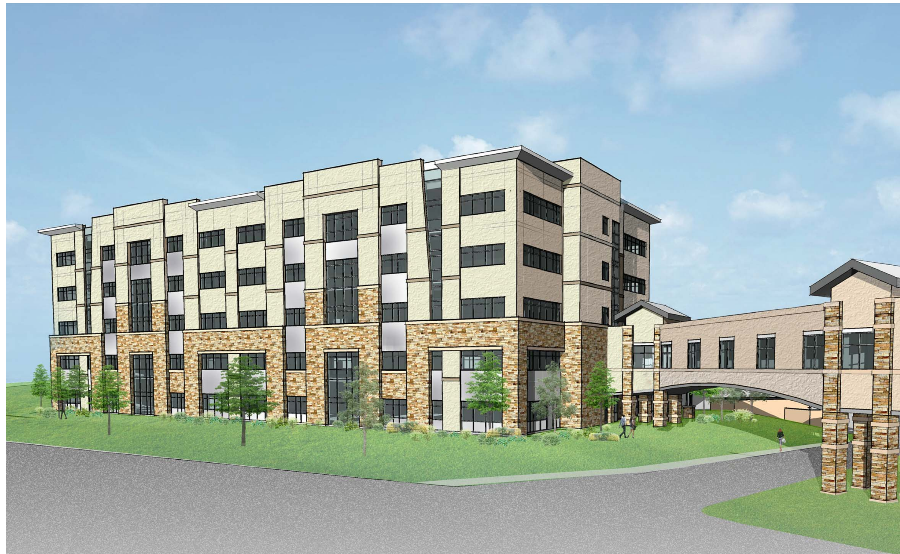
2 SP6 VIEW FROM NORTHWEST
