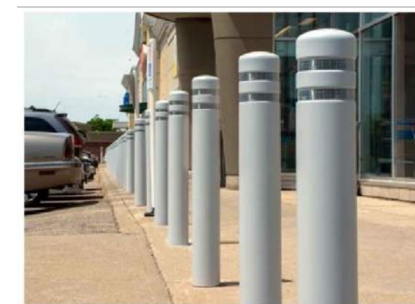
VEHICULAR PROTECTION BOLLARD LEGEND:
