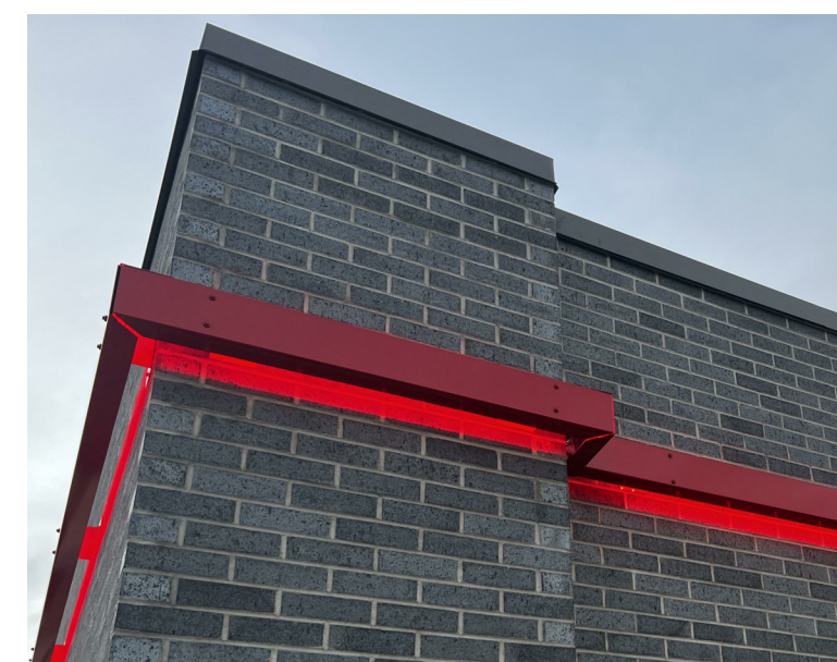
BACK-LIT BANDING; REF TR-1 FOR COLORS NOTE: PHOTO IS INTENDED TO DISPLAY THE RED BANDING AND LIGHT SOURCE AND NOT REPRESENT THE BUILDING MATERIALS FOR THIS PROJECT LOCATION AS CHANGES MAY OCCUR AS REQ'D PER THE LOCAL AHJ.
