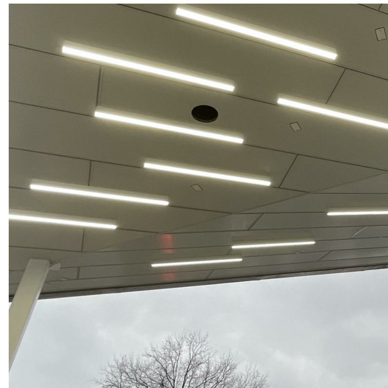
SURFACE MOUNTED LED CANOPY LIGHT FIXTURE: NOTE: PHOTO IS INTENDED TO DISPLAY THE LIGHT FIXTURE AND NOT REPRESENT THE BUILDING MATERIALS FOR THIS PROJECT LOCATION AS CHANGES MAY OCCUR AS REQ'D PER THE LOCAL AHJ.
