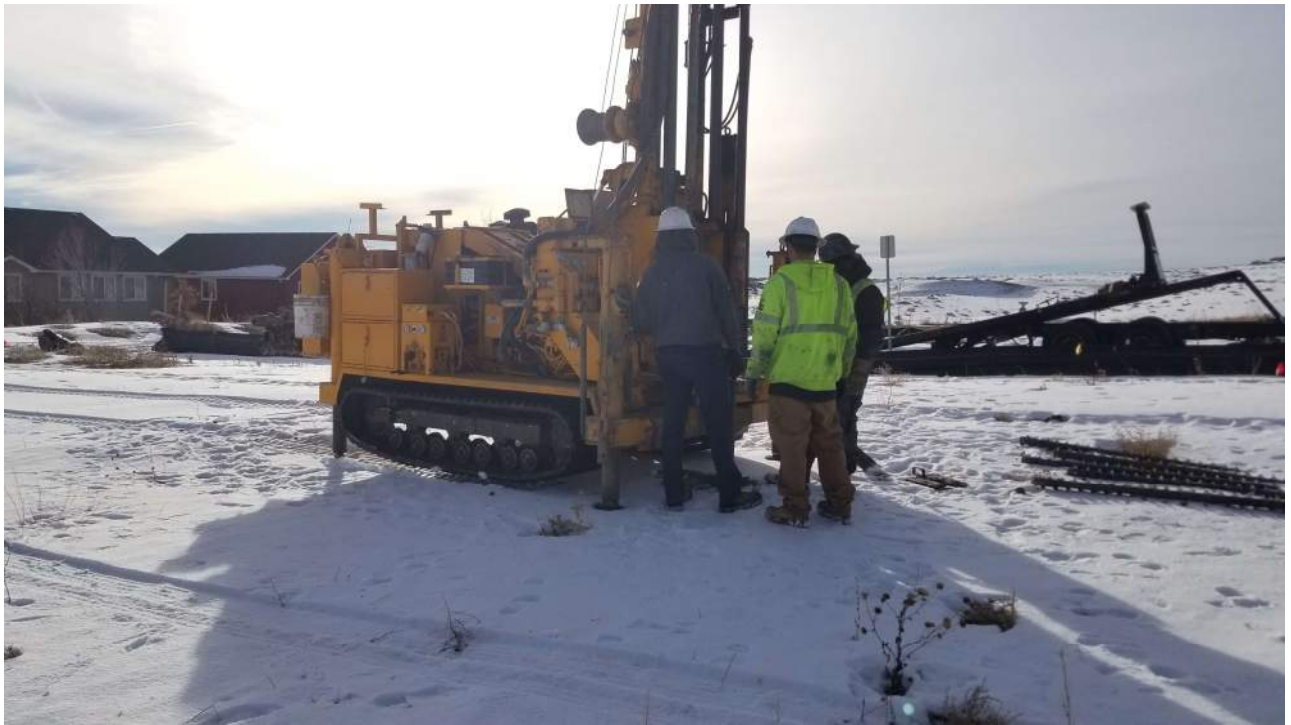
BORING B-5, LOOKING SOUTHEAST
