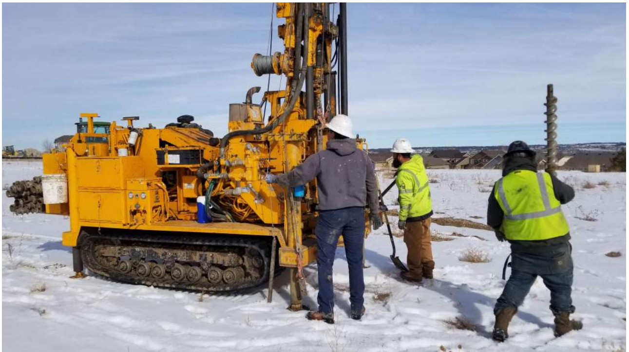
BORING B-2, LOOKING NORTHEAST
