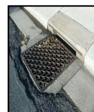
Reticuline Riveted Grate
