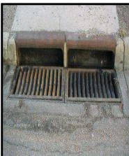
Directional Cast Vane Grate
