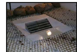
CDOT Type D Inlet Parallel (30° Incline & Depressed)
