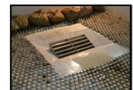
CDOT Type D Inlet Parallel (20° Incline & Depressed)
