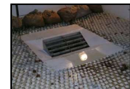
CDOT Type D Inlet Parallel (30° Incline & Depressed)
