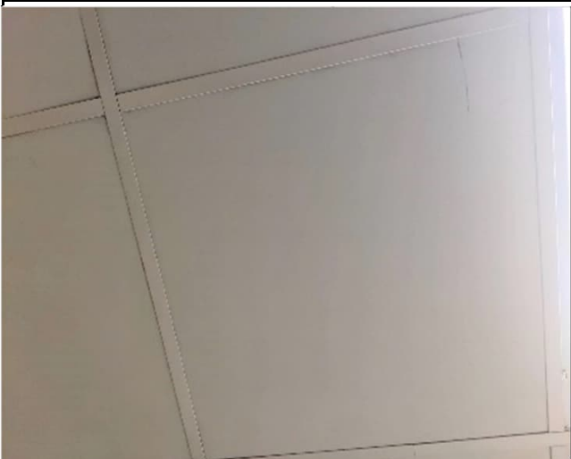
HA# 09 White Smooth 2'x2' Ceiling Tile (Gypsum Board)
