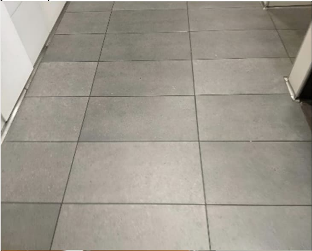
HA# 11 Mortar associated with Ceramic Floor Tile
