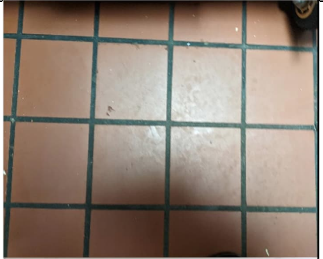
HA# 08 Mortar associated with Red 6"x6" Ceramic Floor Tile
