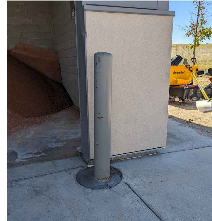
4 BOLLARD EXAMPLE IMAGE - LOADING DOCK AND SHED (COLOR TBD) 09 of 25 NO SCALE
