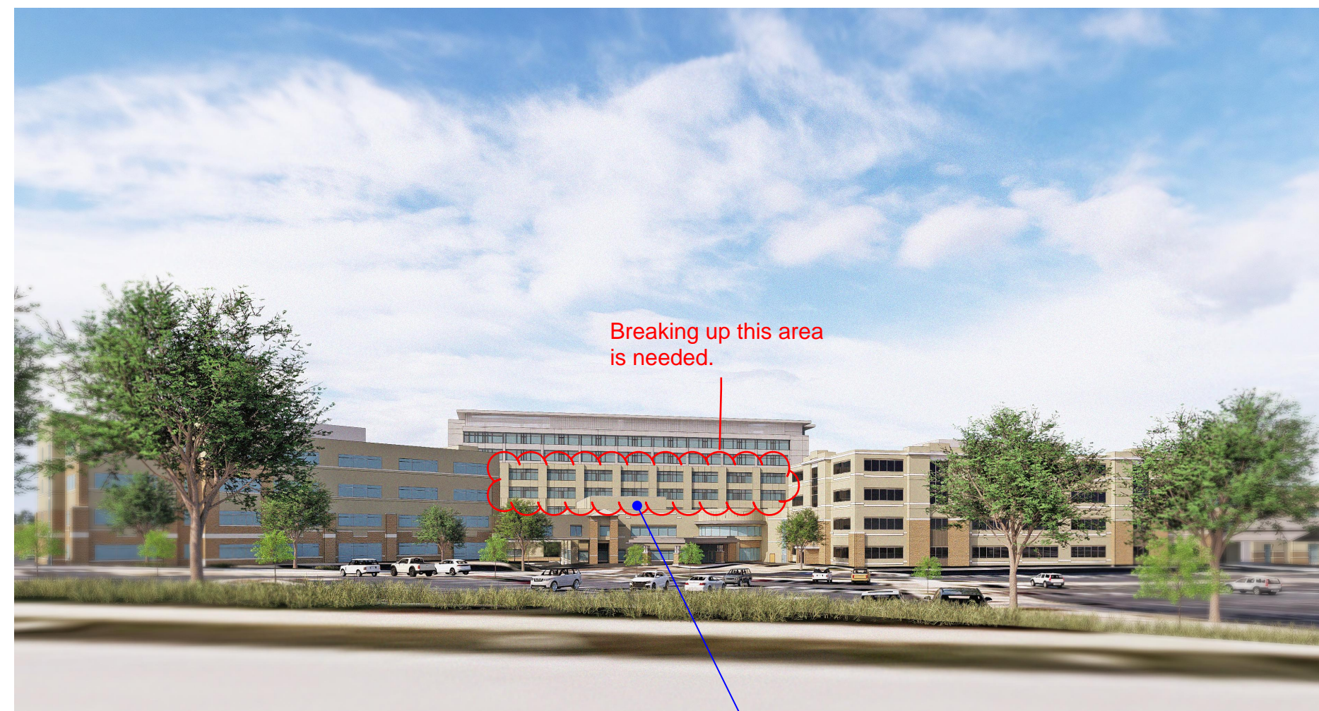
VIEW FROM NORTH
