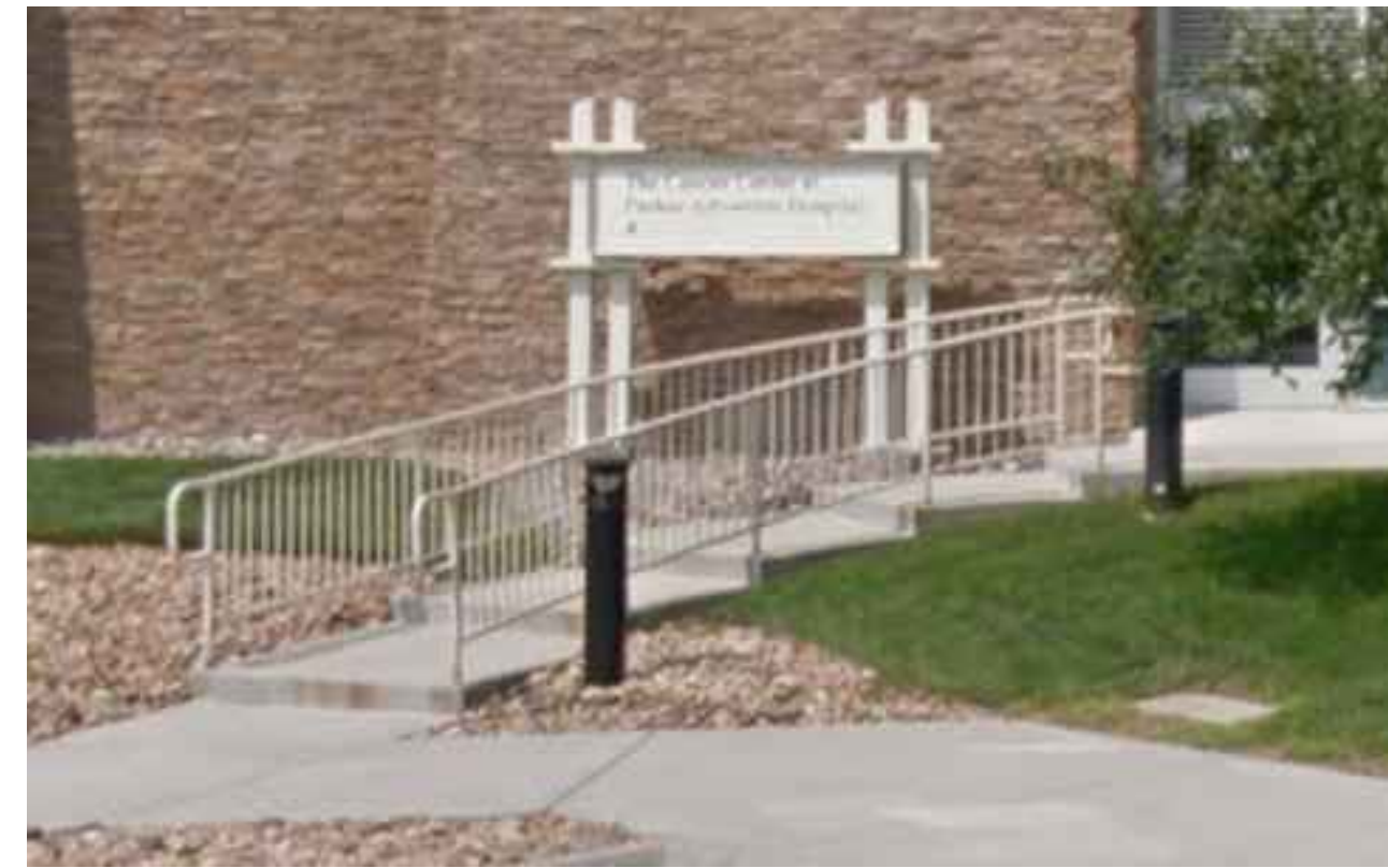
7 MATERIAL: STEEL COLOR: LIGHT GRAY TO MATCH EXISTING HANDRAIL EXAMPLE IMAGE 09 of 25 NO SCALE
