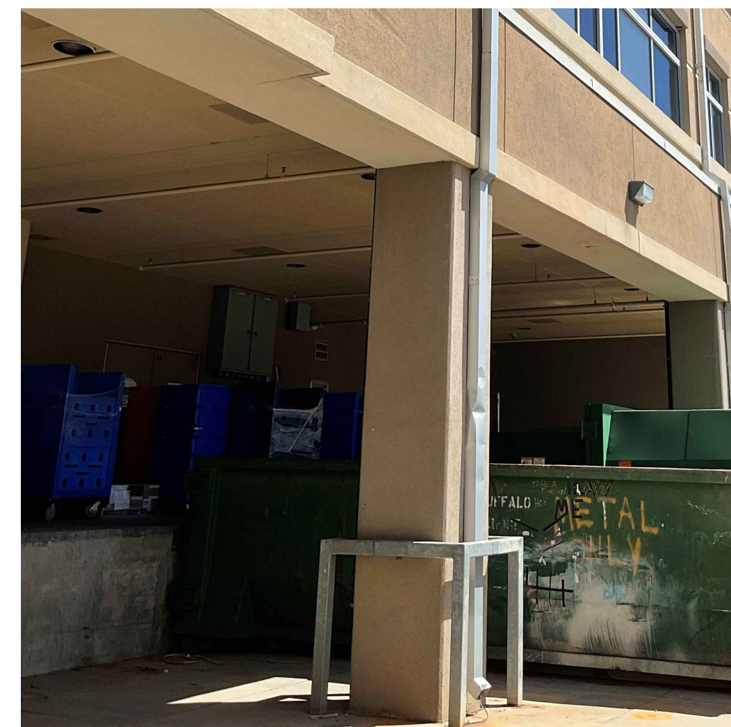
8 MATERIAL: STEEL COLOR: LIGHT GRAY TO MATCH EXISTING COLUMN GUARD EXAMPLE IMAGE 09 of 25 NO SCALE
