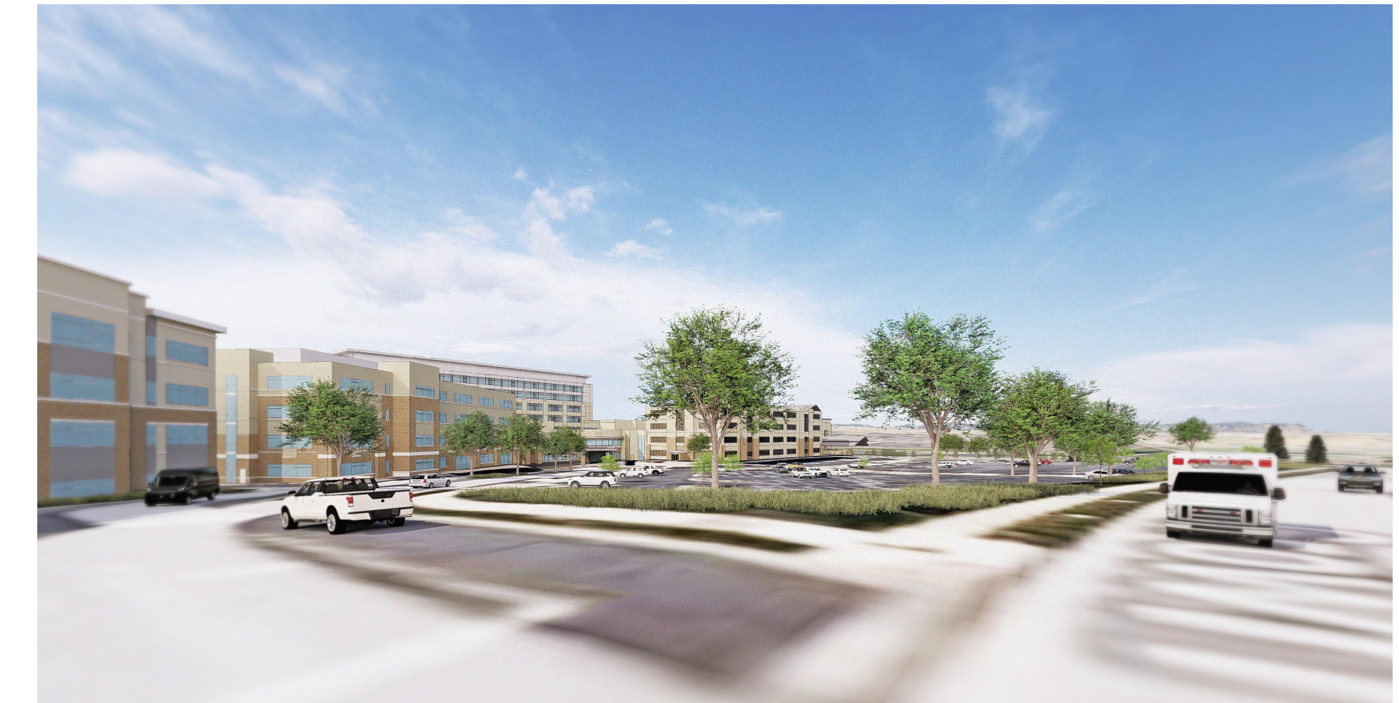
VIEW FROM NORTHEAST
