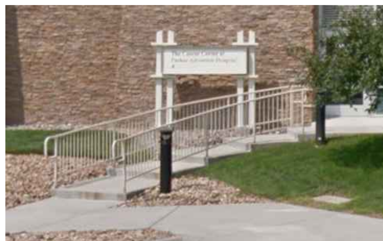
8 HANDRAIL EXAMPLE IMAGE MATERIAL: STEEL COLOR: LIGHT GRAY TO MATCH EXISTING 09 of 25 NO SCALE
