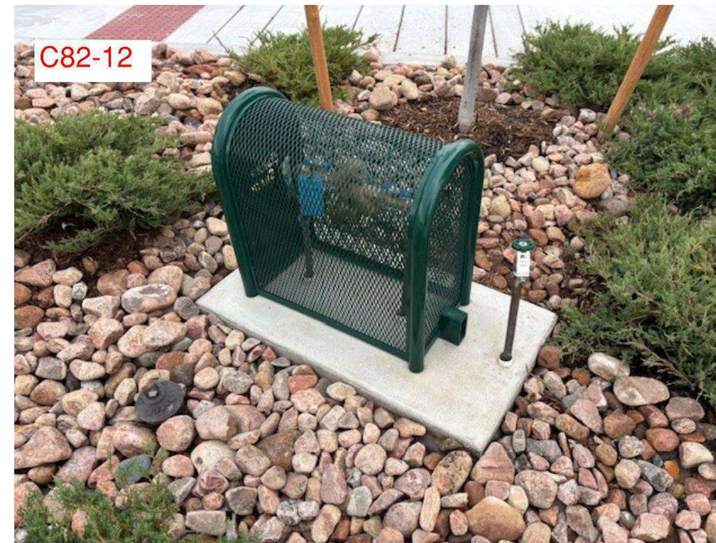
12 IRRIGATION VALVE COVER 1/8" = 1'-0"
