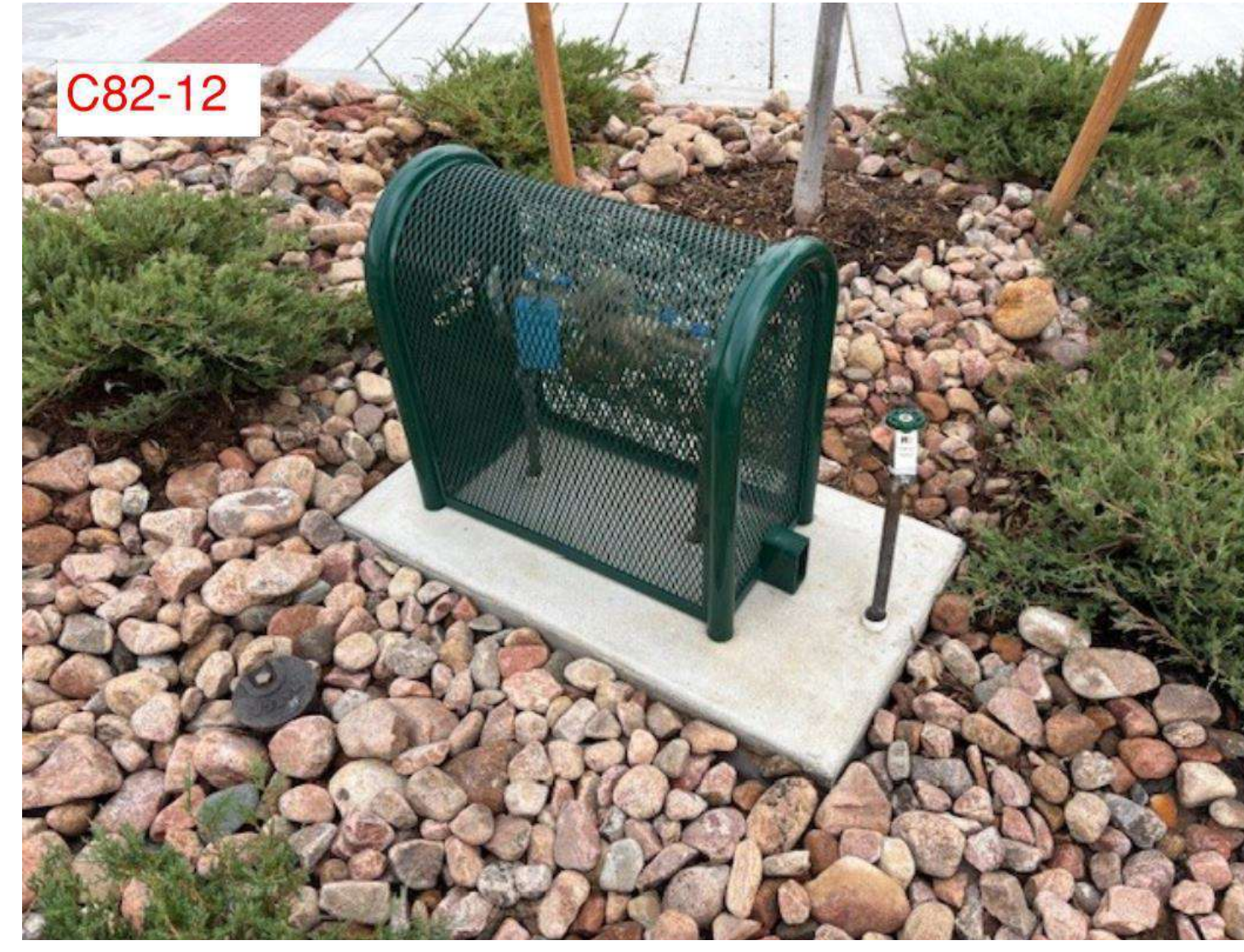
12 IRRIGATION VALVE COVER 1/8" = 1'-0"
