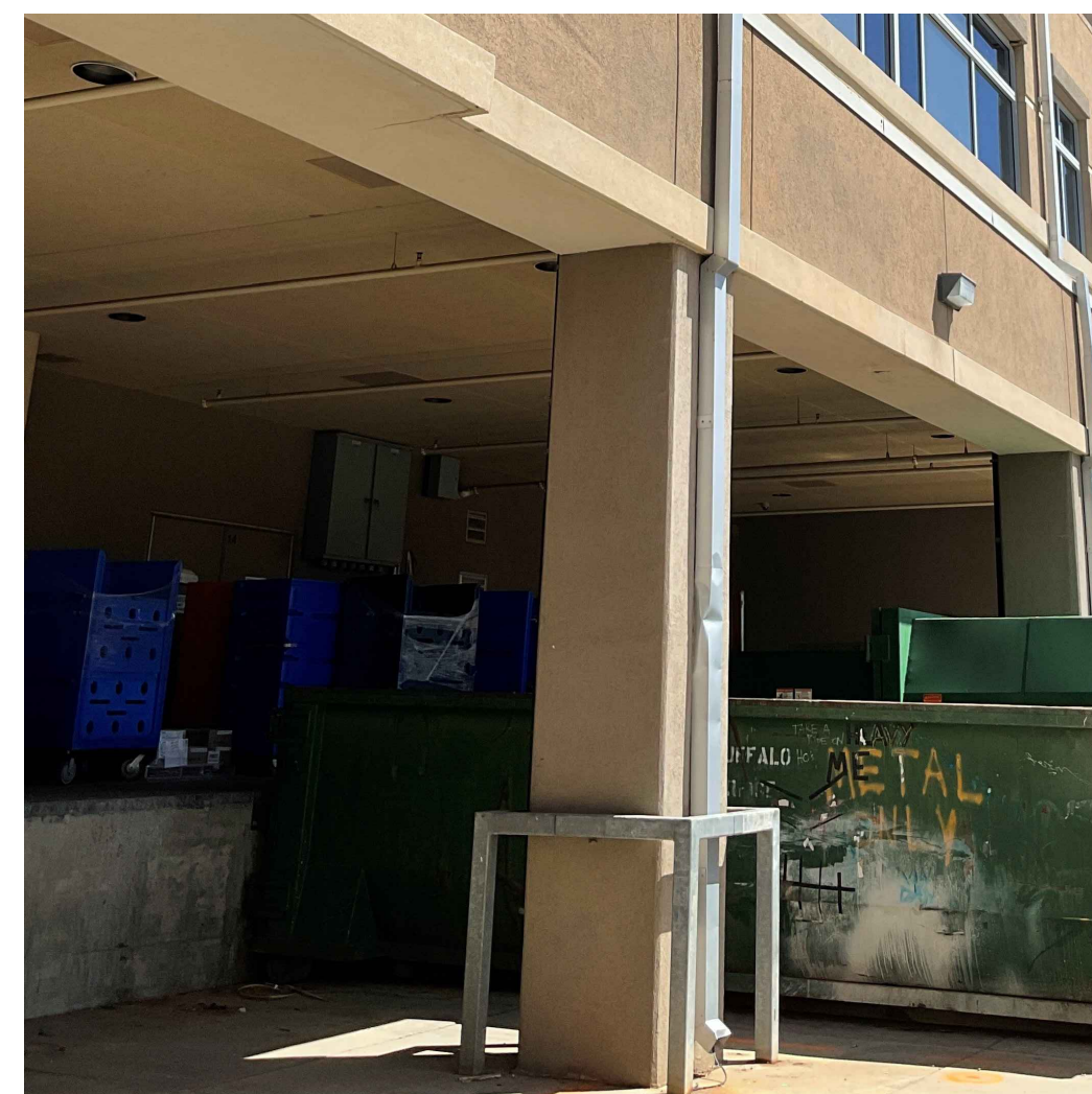
7 COLUMN GUARD EXAMPLE IMAGE MATERIAL: STEEL COLOR: LIGHT GRAY TO MATCH EXISTING 09 of 25 NO SCALE
