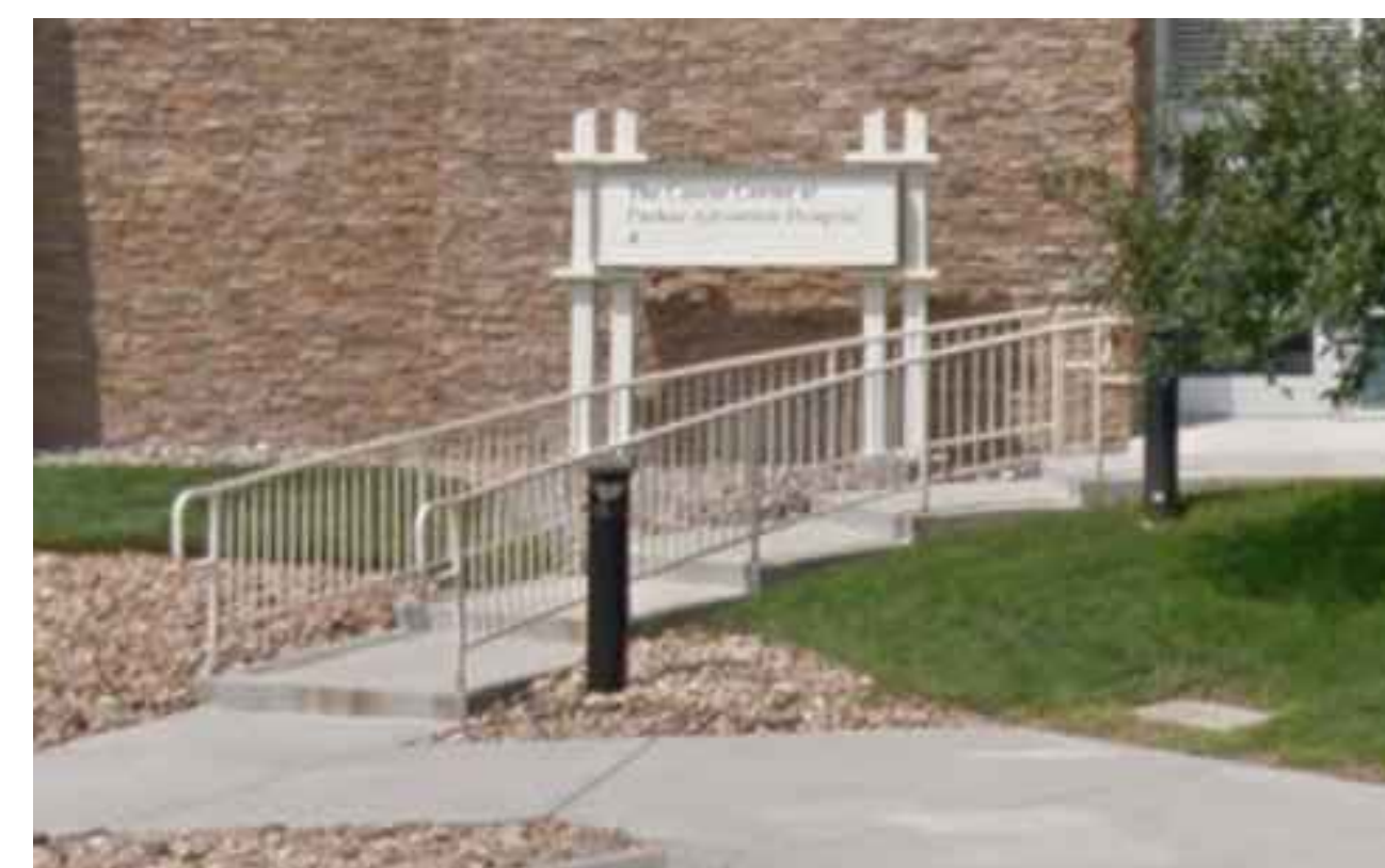
8 HANDRAIL EXAMPLE IMAGE MATERIAL: STEEL COLOR: LIGHT GRAY TO MATCH EXISTING 09 of 25 NO SCALE
