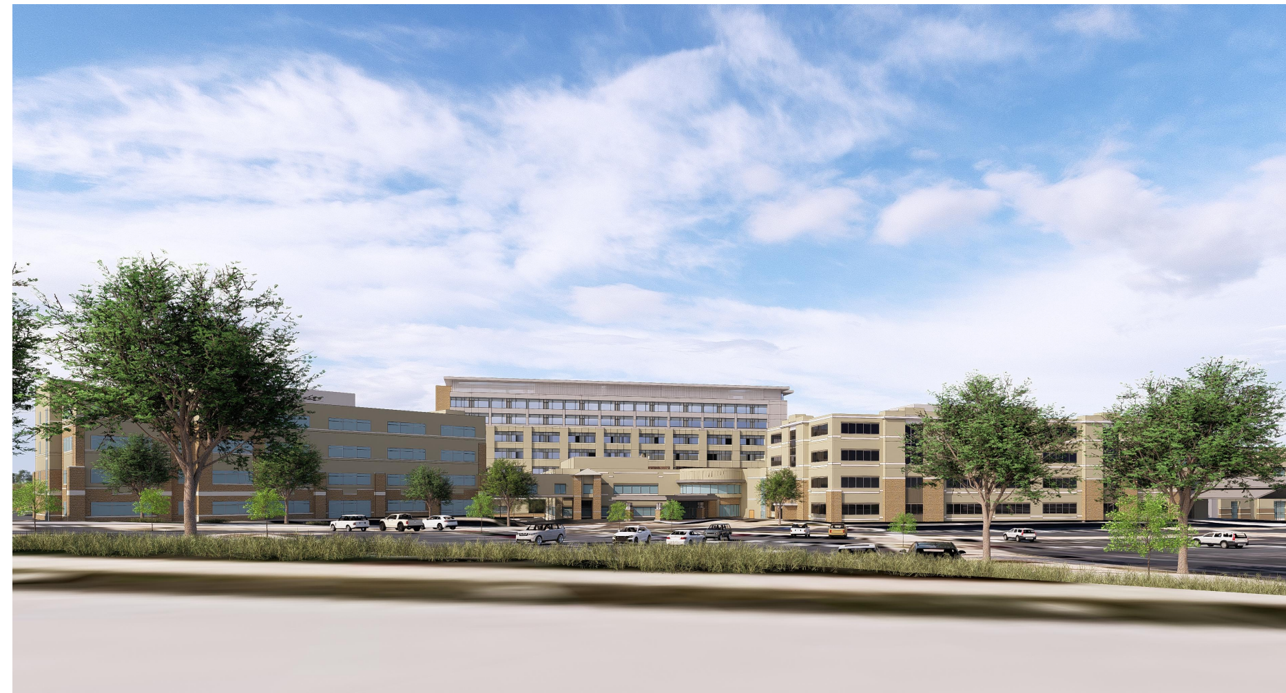
VIEW FROM NORTH
