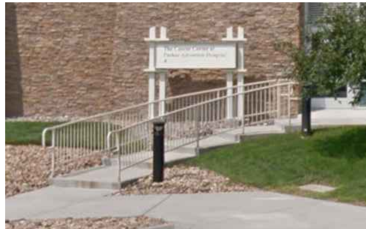
8 HANDRAIL EXAMPLE IMAGE MATERIAL: STEEL COLOR: LIGHT GRAY TO MATCH EXISTING NO SCALE
