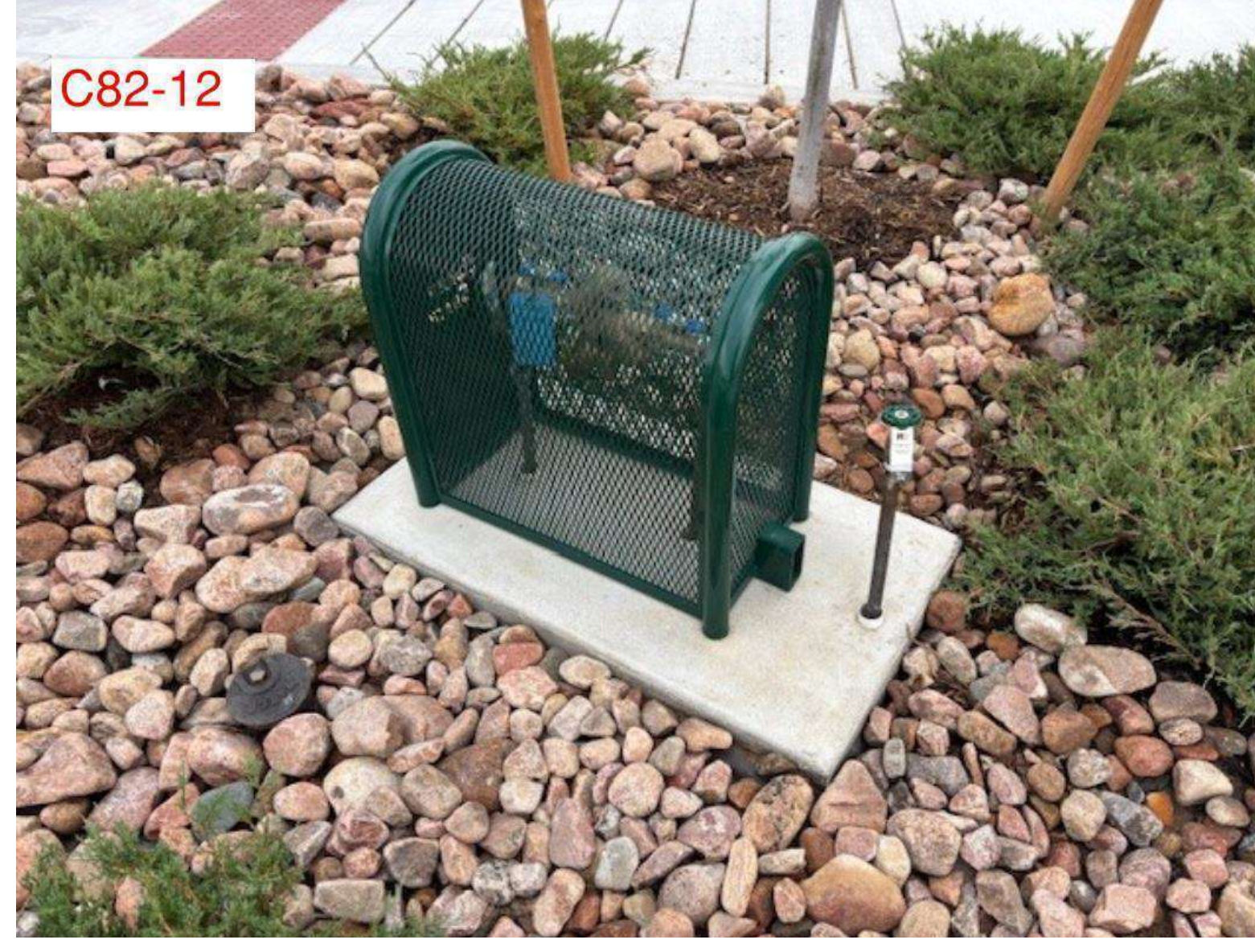
12 IRRIGATION VALVE COVER 1/8" = 1'-0"
