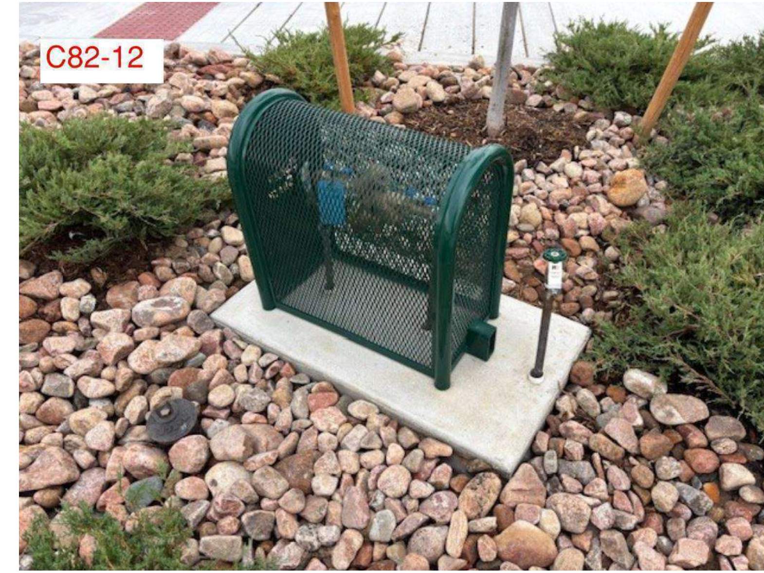
12 IRRIGATION VALVE COVER 1/8" = 1'-0"
