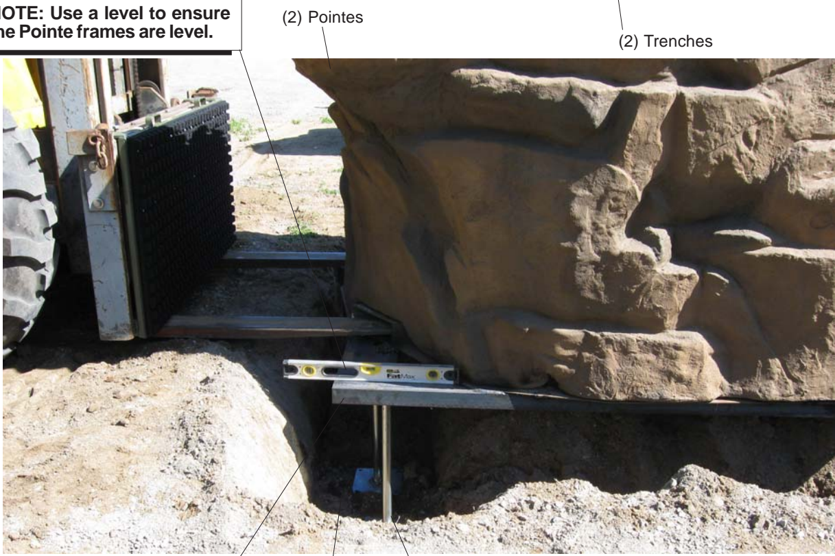
(2) Pointes (2) Trenches (2) Frames (4) Support Braces (2) Trenches
