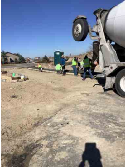
Curb and Gutter on SE corner of Red Sky Road Roundabout
