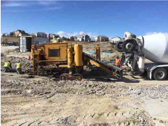
Concrete placement and finishing.
