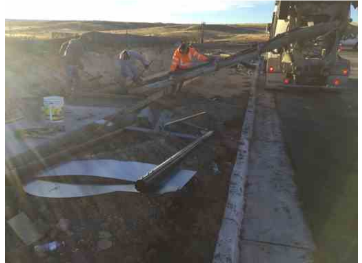
Sidewalk placement
