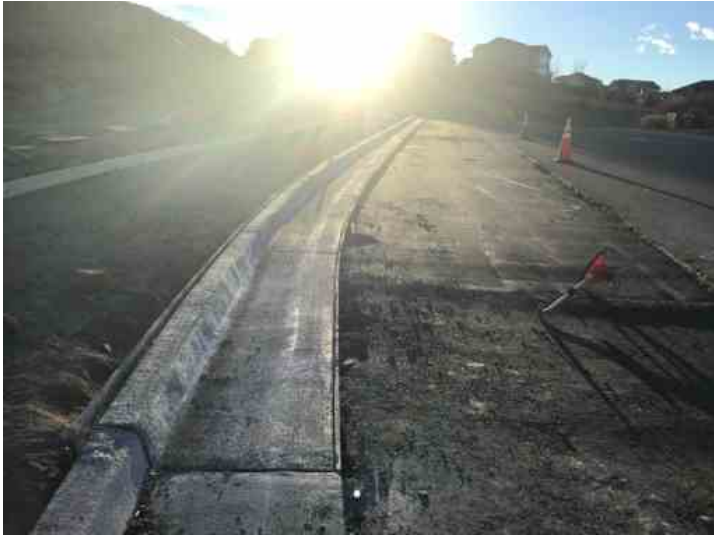
Curb and Gutter along Red Sky Dr
