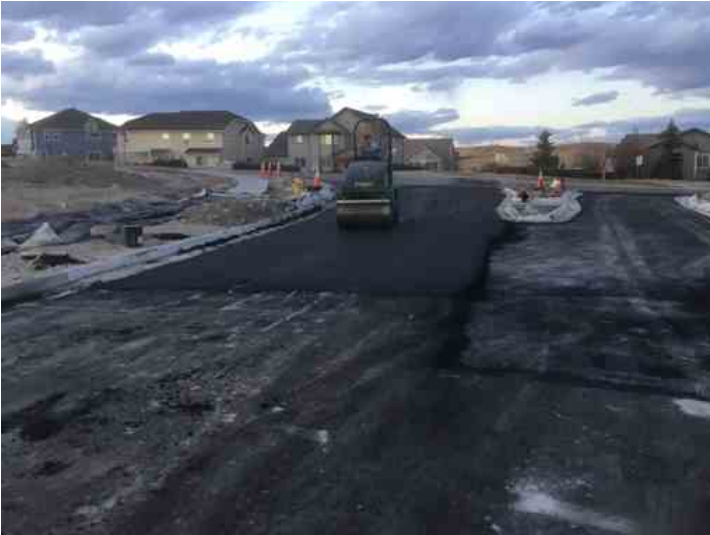
Asphalt being compacted
