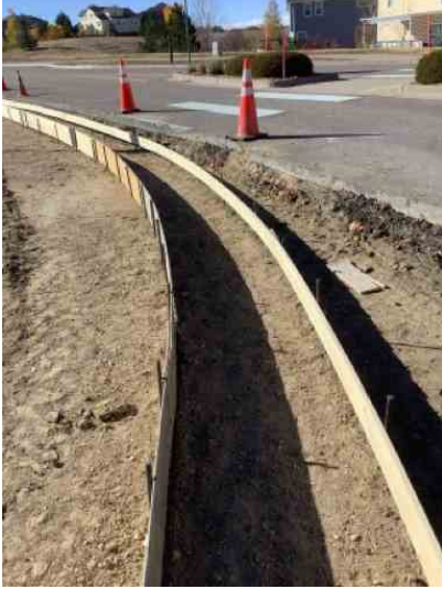
Curb and Gutter subgrade
