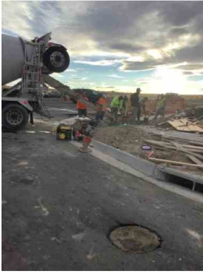
Pouring the ADA Ramp and hand finishing
