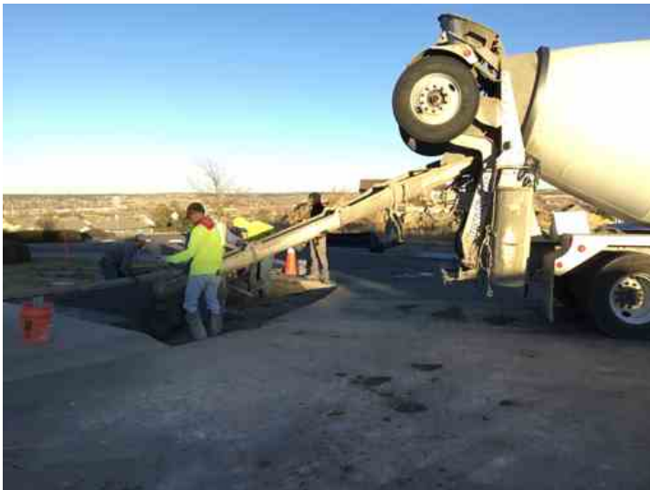
View of concrete placement and delivery method
