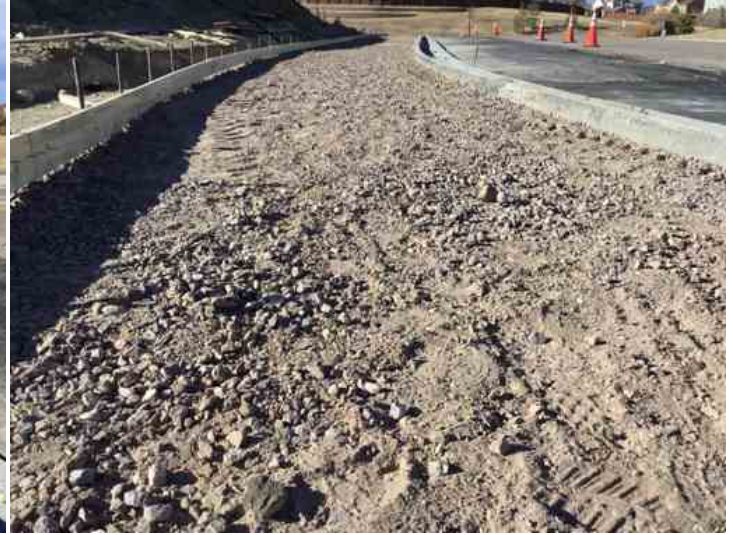
East end of NW sidewalk along South Red Sky Drive
