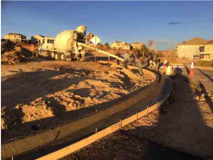
Concrete placement and finishing.
