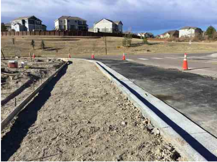
View of subgrade testing (west end)
