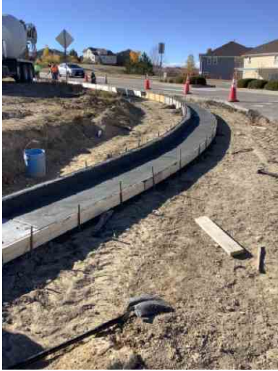
Curb and Gutter on Red Sky Rd roundabout
