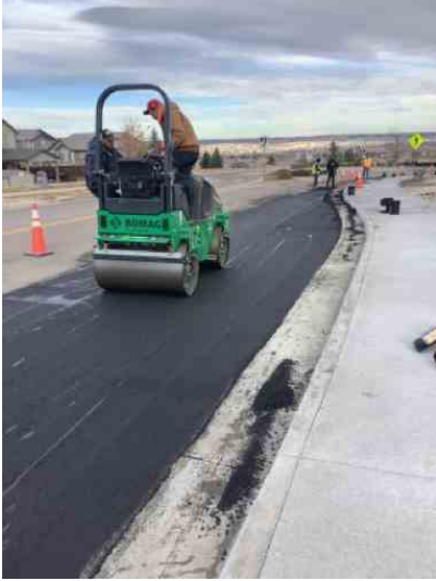
Red Sky Road paving
