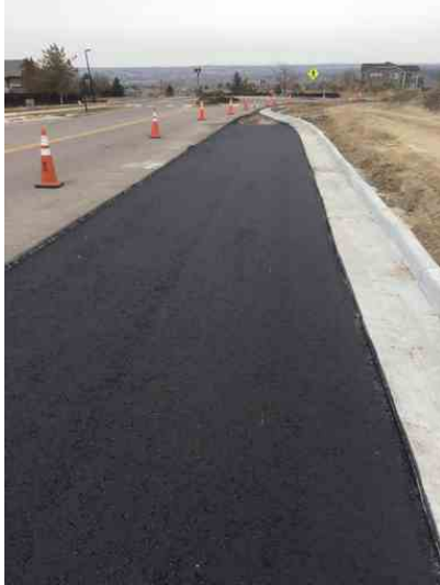
Asphalt placed
