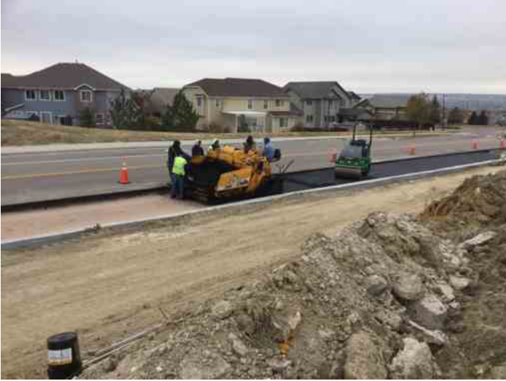
Asphalt being placed.
