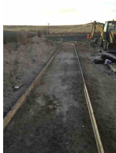
Sidewalk subgrade
