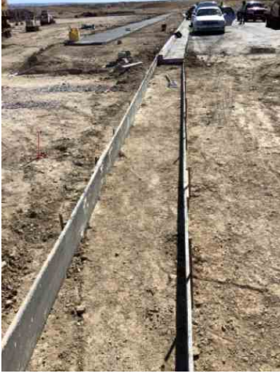
Curb and Gutter subgrade
