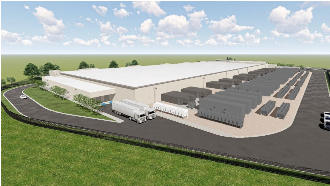
View of the rear loading dock and equipment yard from the CORE substation
