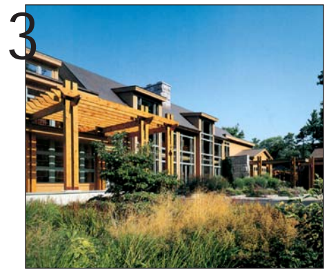
3. Locate front doors facing the street and be accessible from a public sidewalk or pathway. Clearly define, articulate and orient building entrances to pedestrians first, then vehicles.
