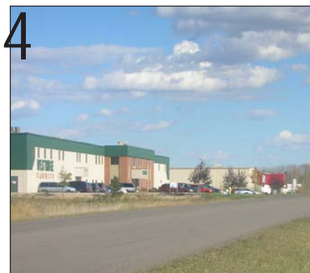
4. Locate buildings close to the main street. Buildings along a street should follow the same 'build to' line with some variances to provide for pocket setbacks, interest and definition.
