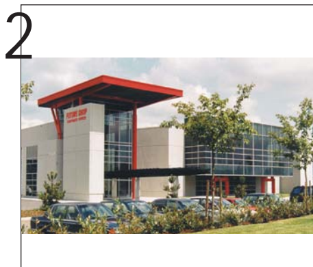
2. Reduce building massing by incorporating different materials, textures or colours, or off-setting portions of the building. (See Land Use Bylaw Sec. 25.4.5)
