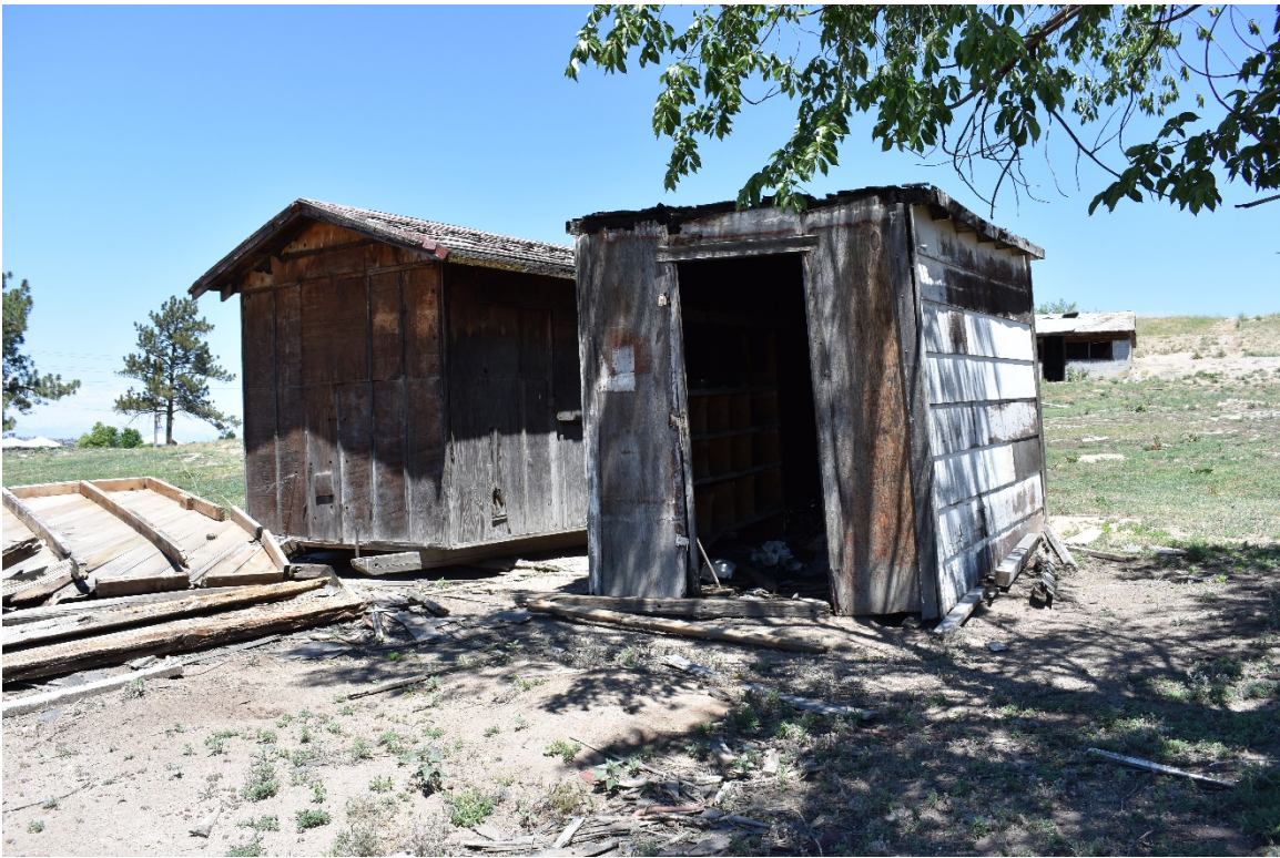
5DA875 – Overview of outbuildings F8 and F9; view to the northwest.
