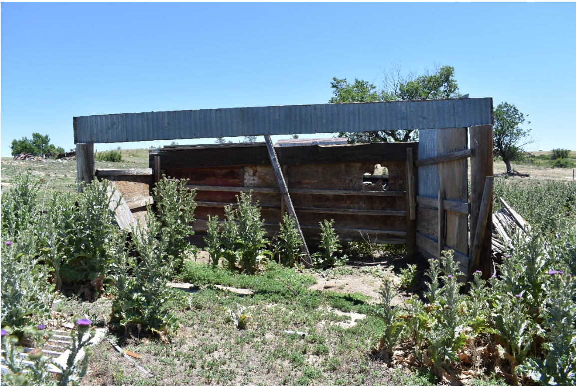
5DA875 – Loafing shed (F7); view to the east. Photograph: DSC_0254 Date: 6/25/2018
