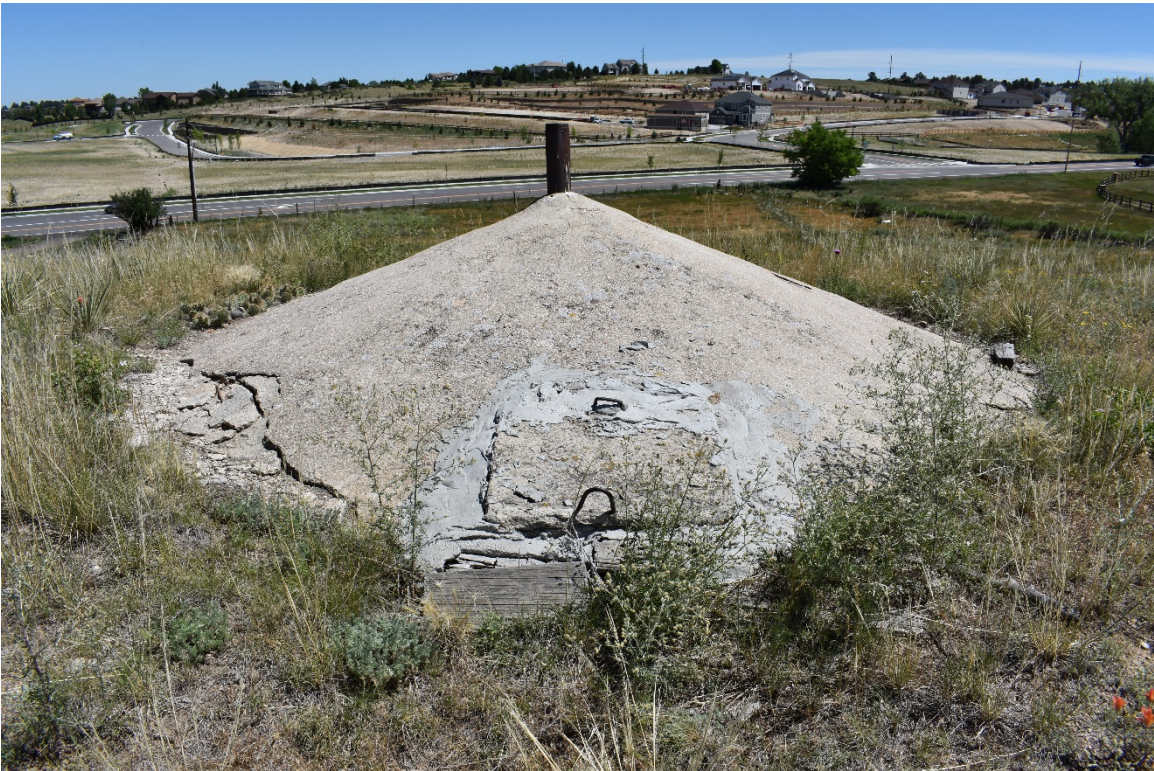
5DA875 – Overview of Cistern (F10) showing door; view to the northwest.
