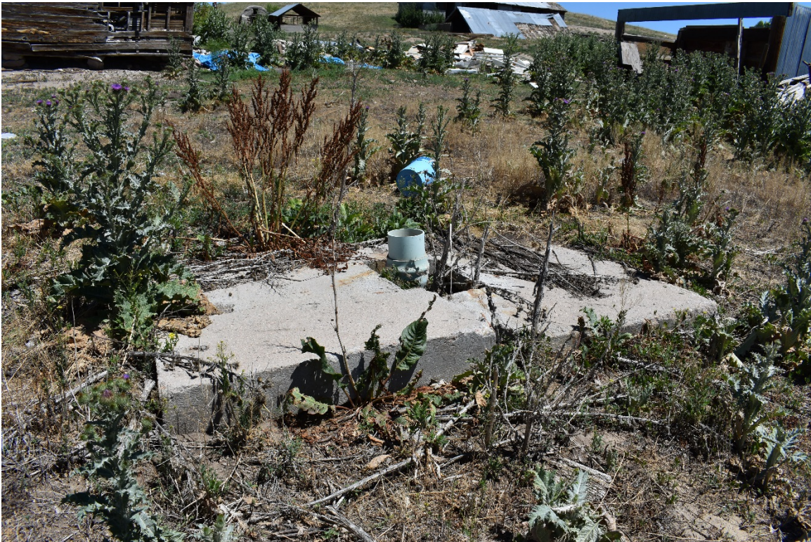
5DA875 – Possible well or cistern (F12) on the south side of house (F1, background); view to the north-northeast. Photograph: DSC_0219 Date: 6/25/2018
